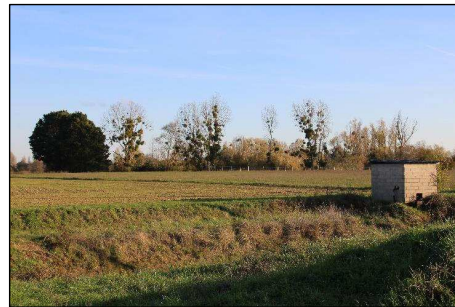
Station de pompage
